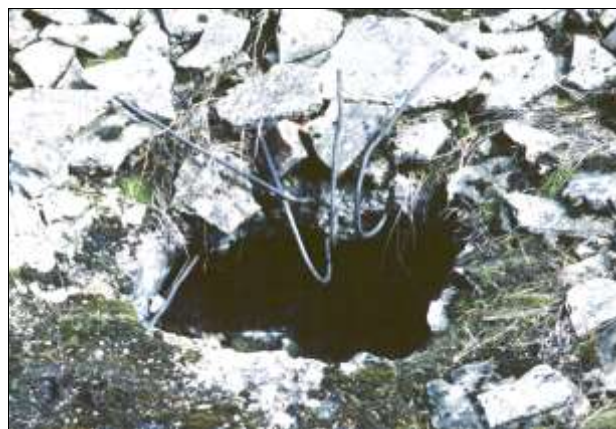
Hole in the shattered roof of Morgue #1 of Crematorium II at Auschwitz-Birkenau. It was created after the war by Polish investigators to gain access to the morgue's interior, because the entry area had collapsed after the building had been dynamited by the Germans before retreating from Auschwitz. Note that the roof's rebar were only bent back, but not removed. (Photo of 1997.)
